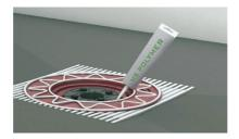
Apply modified thin-set mortar to the floor area including the drain flashing bonding flange except the inner 2-3" area using a 1/8" to 1/4 (3 a 6 mm) V-notched trowel. In order to avoid trapping air under the sheet, trowel mortar in parallel rows across the width or length of the sheet.
