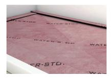
Once you are satisfied with the position of the waterproofing sheet, locate the drain hole by pushing down on the liner. Feel the edges of the drain recess and mark the spot on the WATER-STOP sheet. Remove the sheet from the shower and cut out the marked hole using a utility knife or similar.
