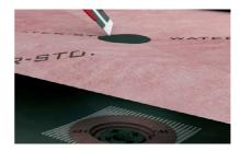
To seal between the drain flashing and the underside of the membrane apply 2 continuous beads of polyurethane or MS sealant separated 2" in concentric circles around the drain hole opening and then a third drop interposed there between in a zig-zagged pattern.
