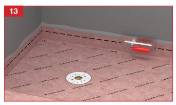
Apply pressure with the flat side of the trowel squeezing the thin-set mortar outward toward the sheet edges in an effort to achieve a 100% bond and coverage, thus eliminating air bubbles and voids between the membrane and substrate (13\*).
