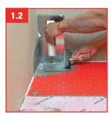
First treat the corners with W-S DIN and W-S DEX inlet and outlet angles.
