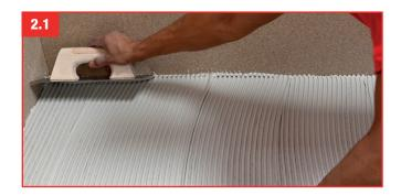
**2.** Apply a suitable adhesive mortar to the substrate. Use a tile adhesive with a minimum classification of C2 according to EN 12004 or ISO 13007 or one that complies with ANSI A118.4, ANSI A118.11 or ANSI A118.15.
