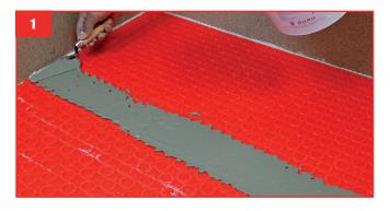
**1.** Apply EASEAL polymeric waterproofing cement centred in a 6" to 8" (15 to 20 cm) wide strip.
