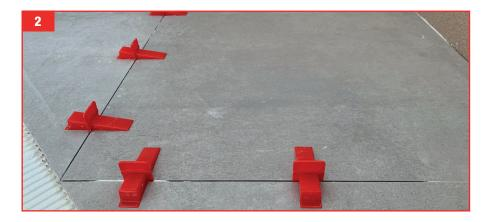
**2.** Lay the tile. Lift a tile frequently to check that the back of the tile is completely covered. Applying a thin layer of adhesive mortar to the back of the tiles is a practical way to achieve adequate coverage.
