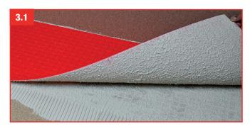
**3.** Place the G-Flex membrane with the white non-woven side over the glue cement and press down firmly with the smooth side of the trowel, a wooden trowel or a roller to achieve full adhesion.
