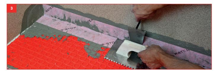
**3.** Place the W-S BAND on the bonding layer. First on the walls and then overlapping at least 2-1/2" (6 cm) over G-Flex. Press with the smooth side of a trowel or spatula to remove air and excess material.
