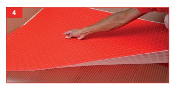
**4.** Then install the following pieces of G-Flex in the same manner. To ensure a flat surface, do not overlap the edges or ends of one membrane over another. Spread G-Flex edge to edge with adjacent pieces without leaving gaps of more than 3 mm between membranes.
