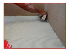
Apply an adhesive mortar suitable for the type of flooring. Use a tile adhesive with a minimum rating of C2 per EN 12004 or ISO 13007 or ANSI A118.4, ANSI A118.11 or ANSI A118.15.
