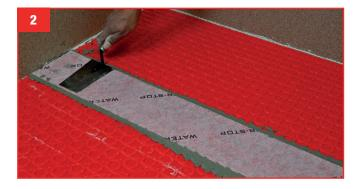
**2.** Place the W-S BAND 14 centred on the joint line and press firmly with the smooth side of the trowel to achieve full adhesion.
