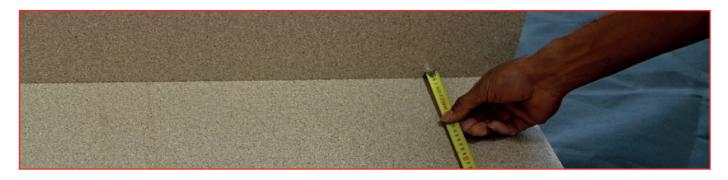
**1.** Cut G-Flex to the required size and shape, leaving a gap of 1/4 inch (5 mm) between the membrane and perimeter walls, columns, architectural elements, structural joints, drains, etc.
